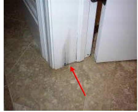
Photo # 60 Pool bath hall door
