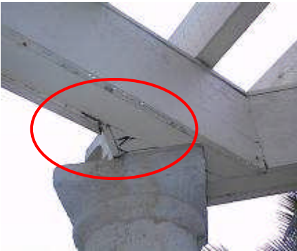
Photo # 55 Wood beams 2 nd fl west
