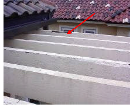
Photo # 54 Wood beams 2 nd fl East
