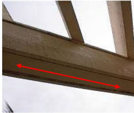
Photo # 53 Wood beams 2 nd fl East
