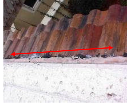
Photo # 51 1 st fl roof line SE
