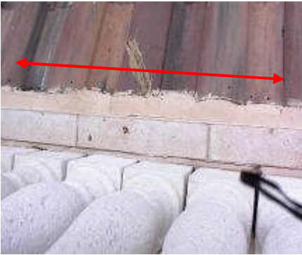
Photo # 52 1st fl roof line SW
